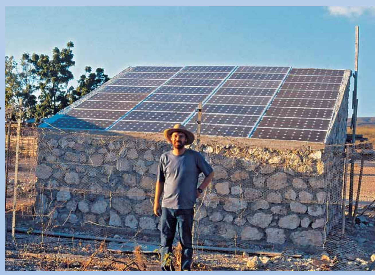
A well with drinking water with 32 solar panels installed on it. Electric power from these solar panels is used for getting water from the depth to the surface. (Haiti)
